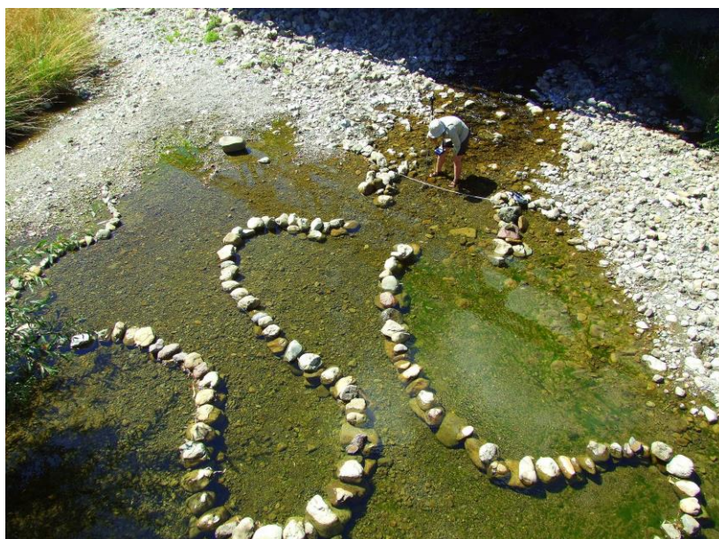
Figure 2a and b: a stable well-defined low-water control section, and b building an artificial low-water control / constriction for gauging low flows
